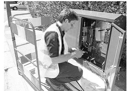
For example, as part of an installation procedure, some companies have the technician check all circuit parameters at the NID before setting up any equipment in the premise. Since this test takes just a couple of minutes as the technician steps through the menu-selected tests, he/she can then move to the location where the equipment will be placed and test the circuit from there.
